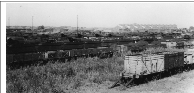
On the Midland & South Western Junction line: a view of the rear of the GWR Works, Swindon. © Ian Watkins
